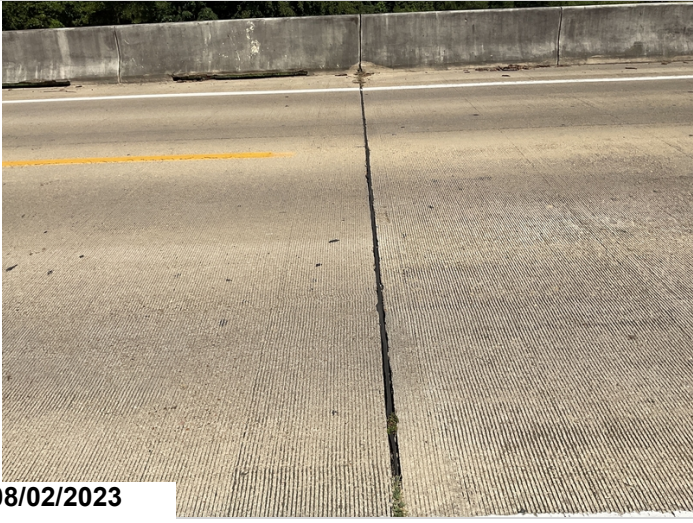
Bent 4, joint material has loss of adhesion.
